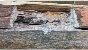
As I stated above, the work is very difficult, but it is progressing close to plan. The demo is going as expected and the process of reinstalling the new tuckpointing is also going as planned. We are encountering some unexpected things in key two areas – the condition of the main stone and conditions at the parapet walls at the top of the tower. Many main stones that were cracked to the point of falling apart.
